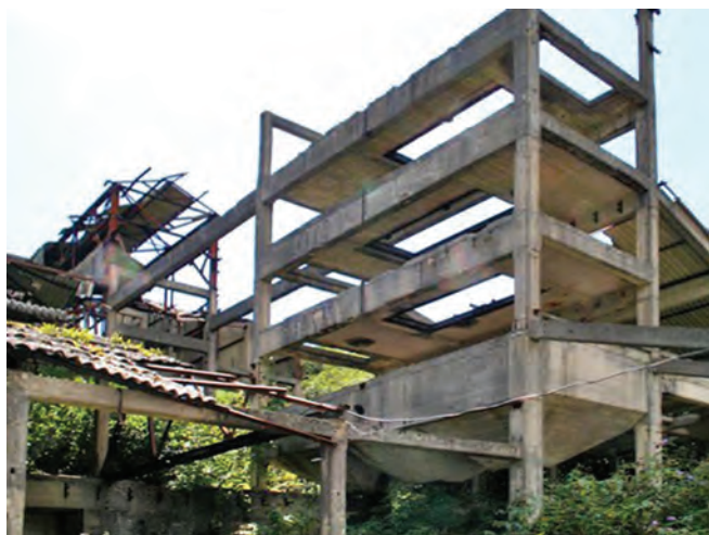
The WWII mill at Hemerdon
